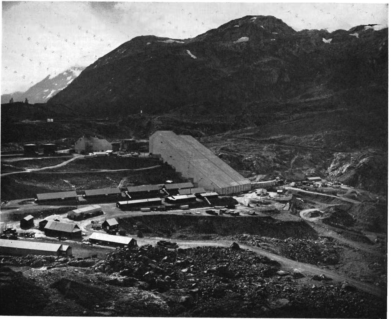
The new 7500-tpd copper concentrator of Granduc Operating Co. receives ore through a 10.3-mile tunnel connecting the mine with the mill at Tide lake, 32 miles by road from Stewart, B.C.
